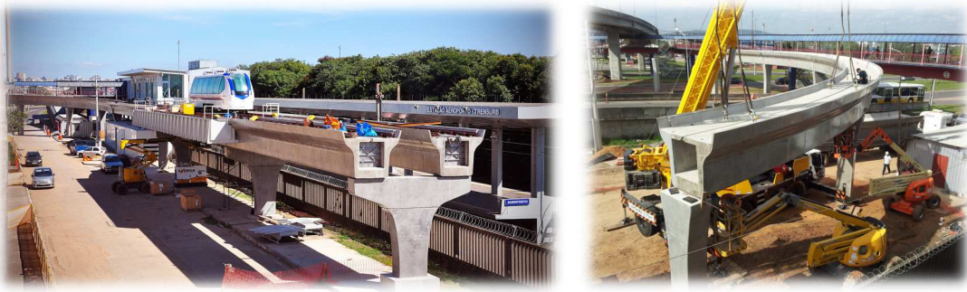
Fig.10 Photos of the construction of the elevated guideway of for Aeromovel.
